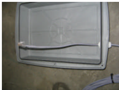
Figure 6. Secure connector to the cable
