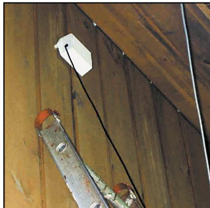
**Figure 4—The Ultimeter Outdoor Humidity and Temperature Sensor must be installed in the shade, where it can never receive direct sunlight. It must also be protected from wind and rain, and in a place that allows air to circulate freely around it.**
