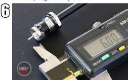
Cut and remove the tape and dieletric for a lenght as illustrated in the caliber (mm).
